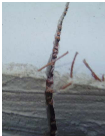
Figure 5: Polymer fibers act as small bridges between the two pieces of the broken panel.
