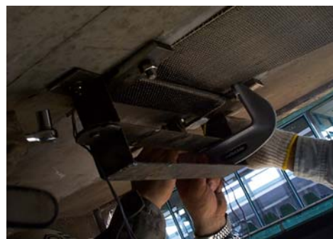
“Fig.13. Buckle and vise type post-tension device.”
