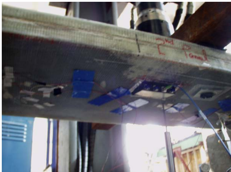
“Fig. 10. Bridge under mechanical fatigue test”
