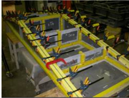
Figure 2 - Fabrication stage showing internal diaphragms
