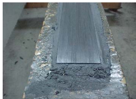
Fig. 3. Beam with the reinforcement
